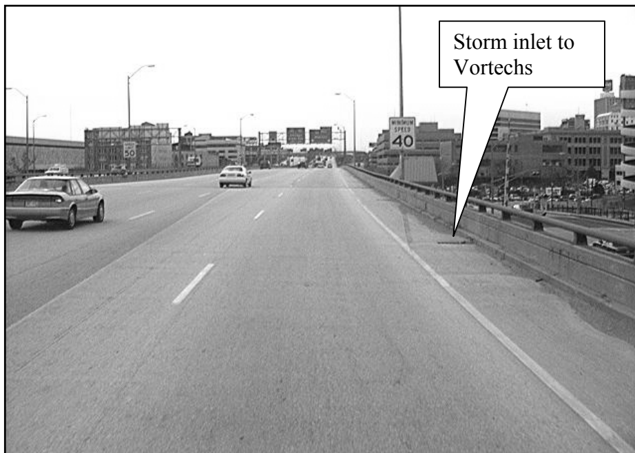
Figure 3-3. Vortechs drainage area condition.
