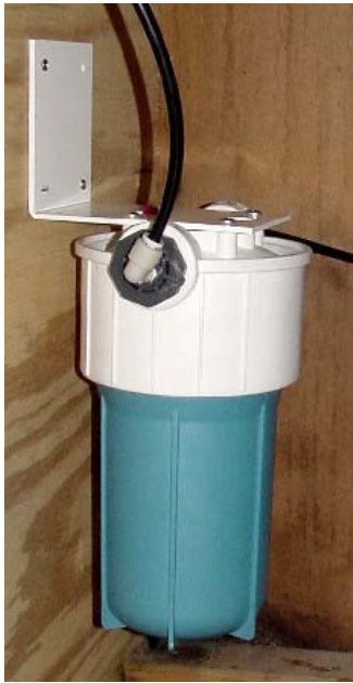
Figure 8. 1-stage POU adsorption system
