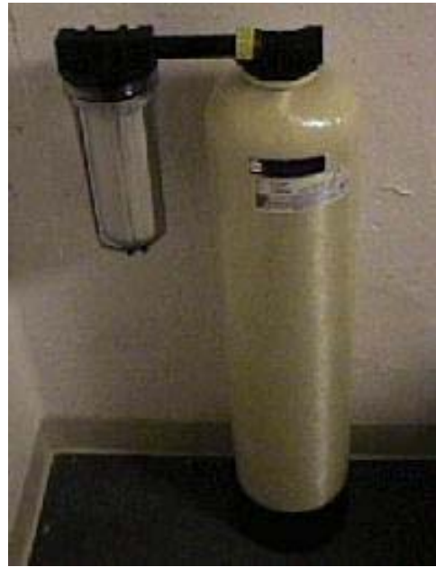
Figure 9. 2-stage POU adsorption system
